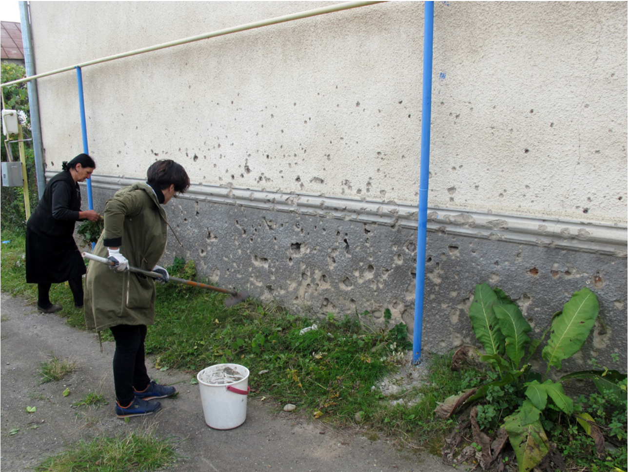
Image 06 Georgian artist Tamar Botchorishvili conducting material tests to repair the bullet holes in the wall of a house in Zemo Nikozi (photo: Sabine Schlatter).
