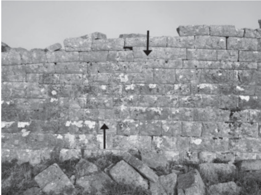
Fig. 5. Stepped joint at the outer face of the curtain between Towers 6 and 7, the arrows marking the start and the end of the steps in the layers (photograph by the author)
