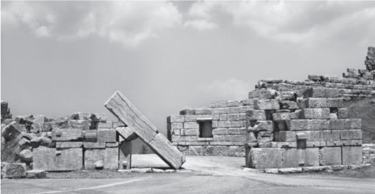
Fig. 6. The Arcadian Gate with its round courtyard, the tilted middle pier of the double entrance, and the decorative consoles facing the town (photograph by the author)
