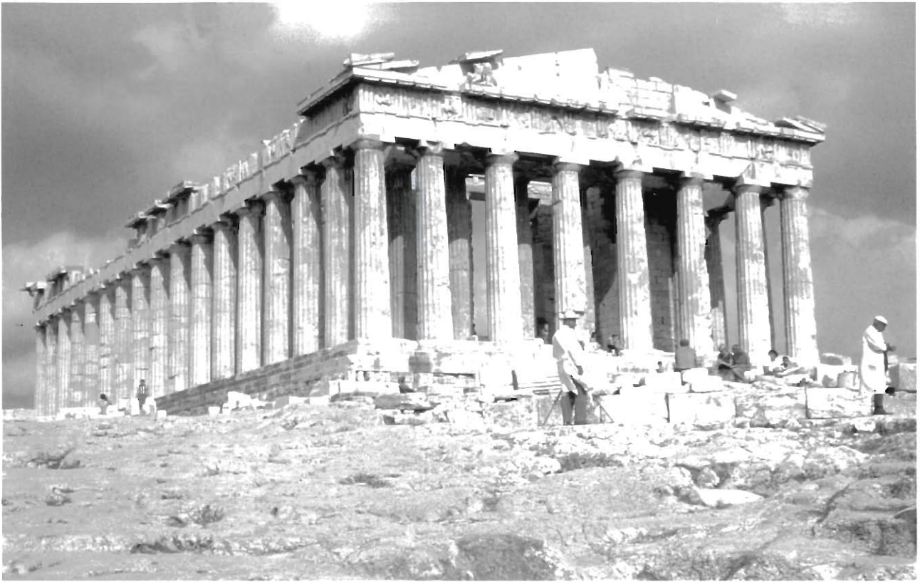
Fig. 9. The Parthenon seen from the Propylaea, in an oblique view to the right.
