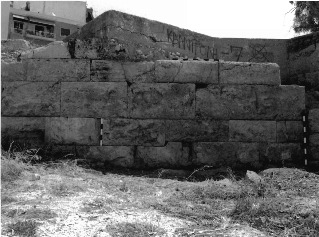
Fig. 16. Peiraiki, P-T1, curtain west of tower P-T1, with polygonal block in lowest course, and blocks with bevelled edges in 4th course from bottom (M.M. Nielsen 2006).
