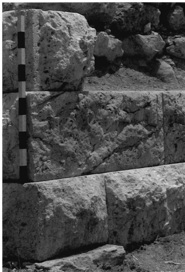
Fig. 20. Peiraiki, Tower P-T1. south western corner with drafted sides (detail of Fig. 11). (M.M. Nielsen 2006).
