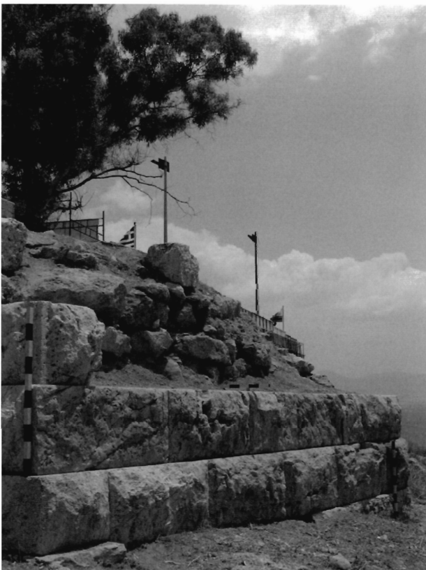
Fig. 17. Peiraiki, P-T1, tower, south face (M.M. Nielsen 2006).
