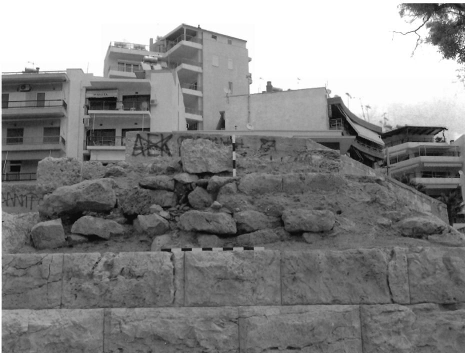
Fig. 22. Peiraiki, P-T1, inner lining with blocks in tower fill, south face (M.M. Nielsen 2006).
