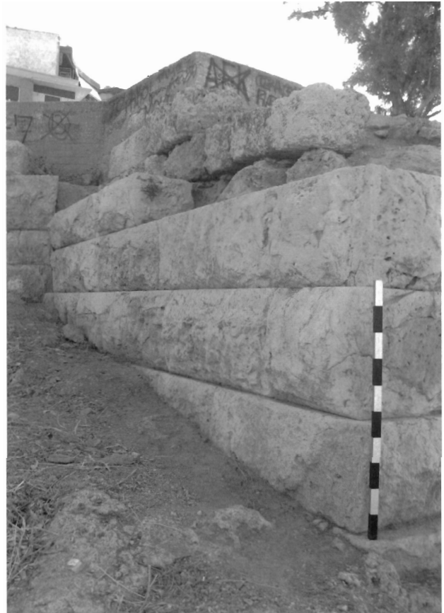
Fig. 23. Peiraiki, P-T1, west face and inner lining with blocks in tower fill (M.M. Nielsen 2006).
