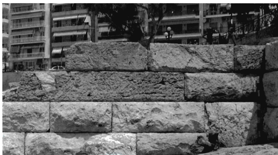
Fig. 19. Peiraiki, P-T2. blocks with beveled edges in tower, east side (detail of Fig. 15) (M.M. Nielsen 2006).
