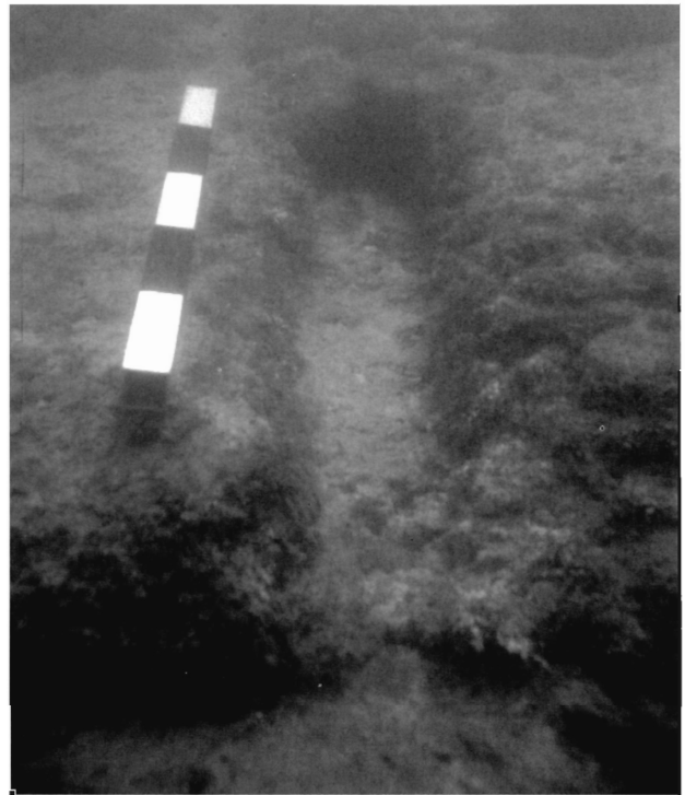
Fig. 4. Slipway 3, rock-cutting for transverse ramp timber. Note the rock-cut foundation trench for the later ramp of Shipshed 10 (Phase 2) in the bottom of the photograph. Heath/©ZHP 2006.
