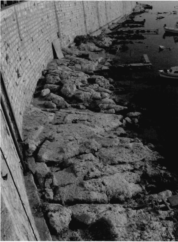
Fig. 7. Area 3, rock-foundations for the fortification wall along the eastern part of the harbour mouth. Nielsen/©ZHP 2006.
