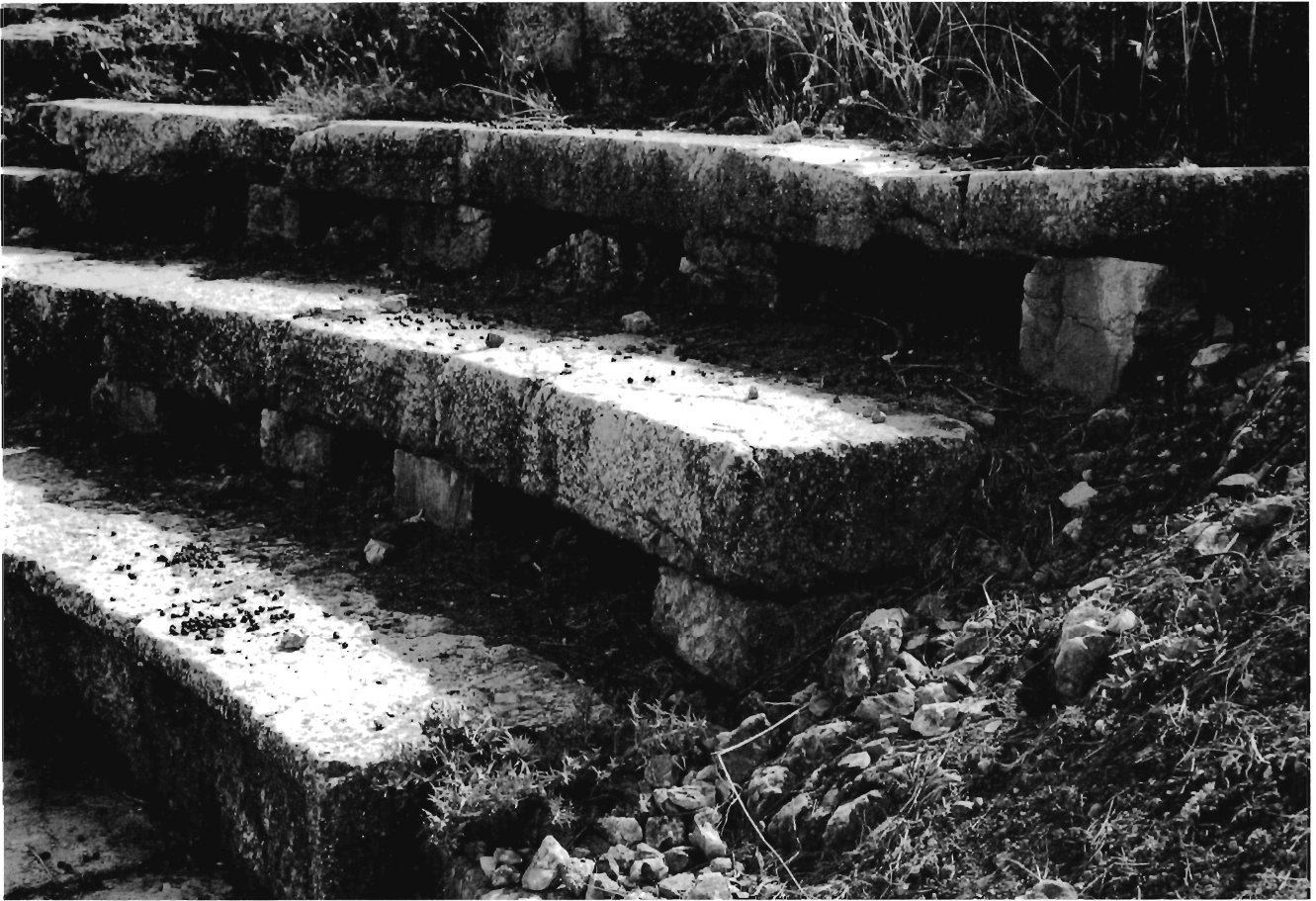
Fig. 11. Orchomenos (Arkadia) from the N. Economical plate-on-block seating combined with simple seating. (Photo: R. Frederiksen)
