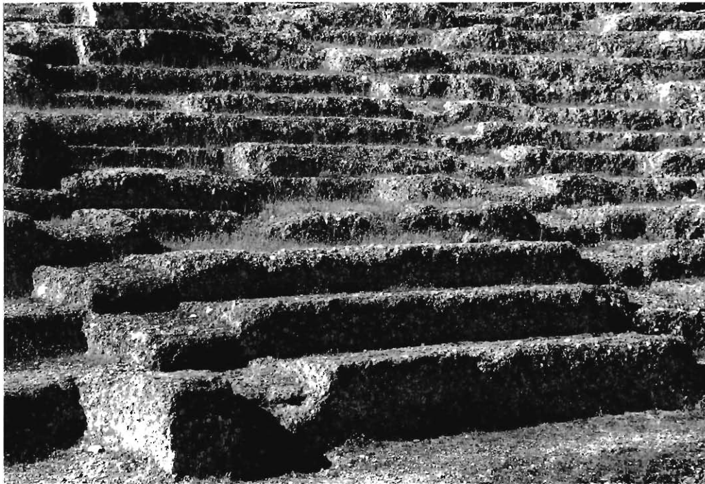
Fig. 2. The theatre at Aigeira from the E. Example of 1:1 relation between steps in stairway and rows of seats. (Photo: R. Frederiksen)
