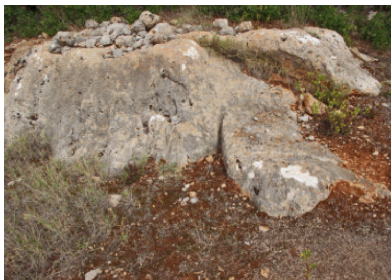
Fig. 58. Section C4. Extensive rockcuttings.
