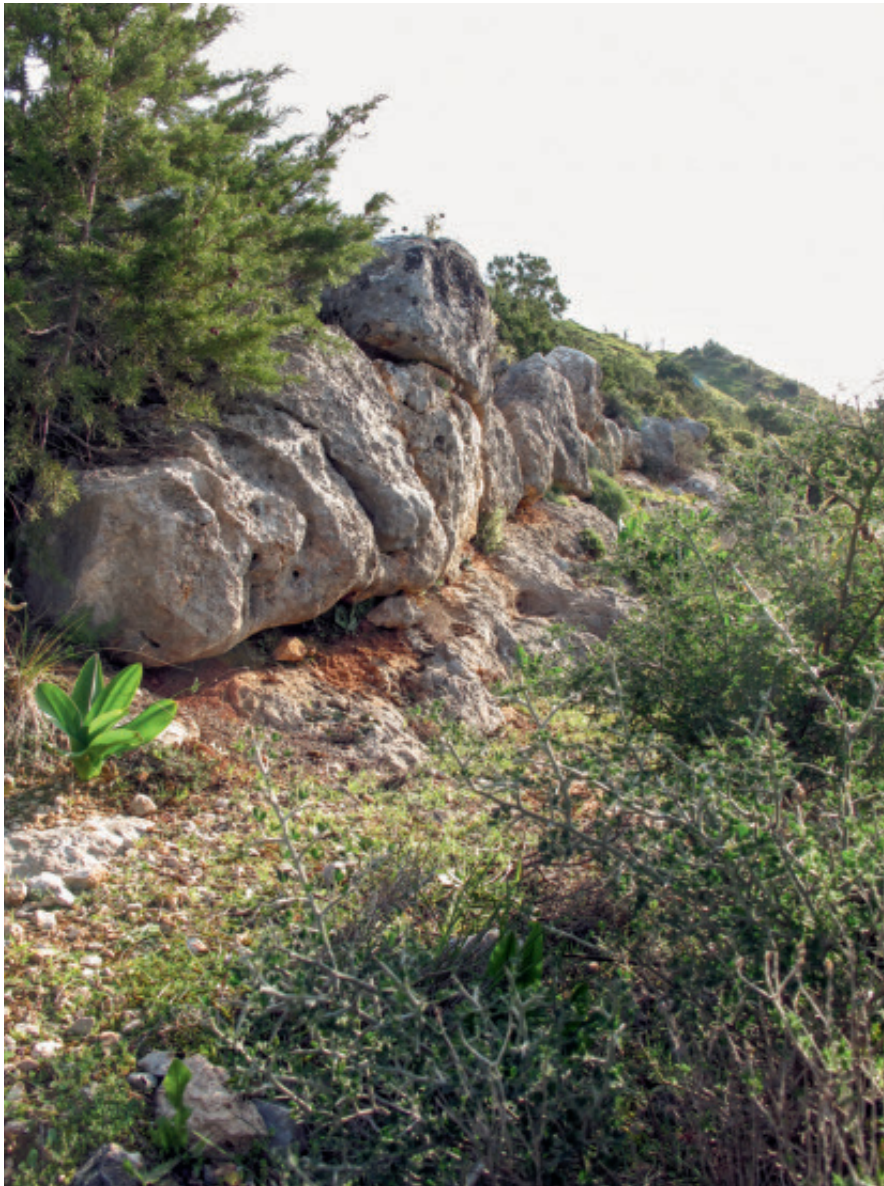
Fig. 13. Stone rows which in some places are made higher with an extra course; the flat façade in this terrace wall is given an even front with coarse adaptation, executed with a sledgehammer and large pointed chisel.
