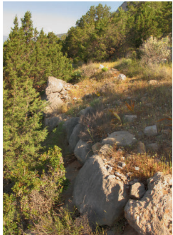
Fig. 37. Remains of a support wall below the track in Area B5b.
