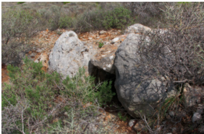
Fig. 43. The outlet, which is possibly a land-drain off the cultivated area, seen from outside the edge
