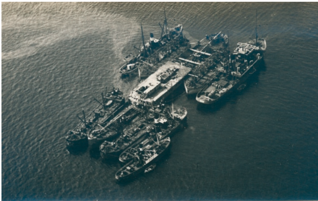
M/S «ESBJERG» salvaged by wreck-raising pontoons in the Baltic during the summer 1946.
