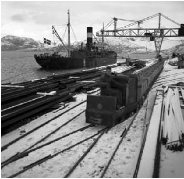
The cryolite quarry at Ivittuut. Greenland's most important raw material, cryolite, was used in aluminium production and was essential to American heavy industry. (Photograph by Jette Bang, the Arctic Institute)
