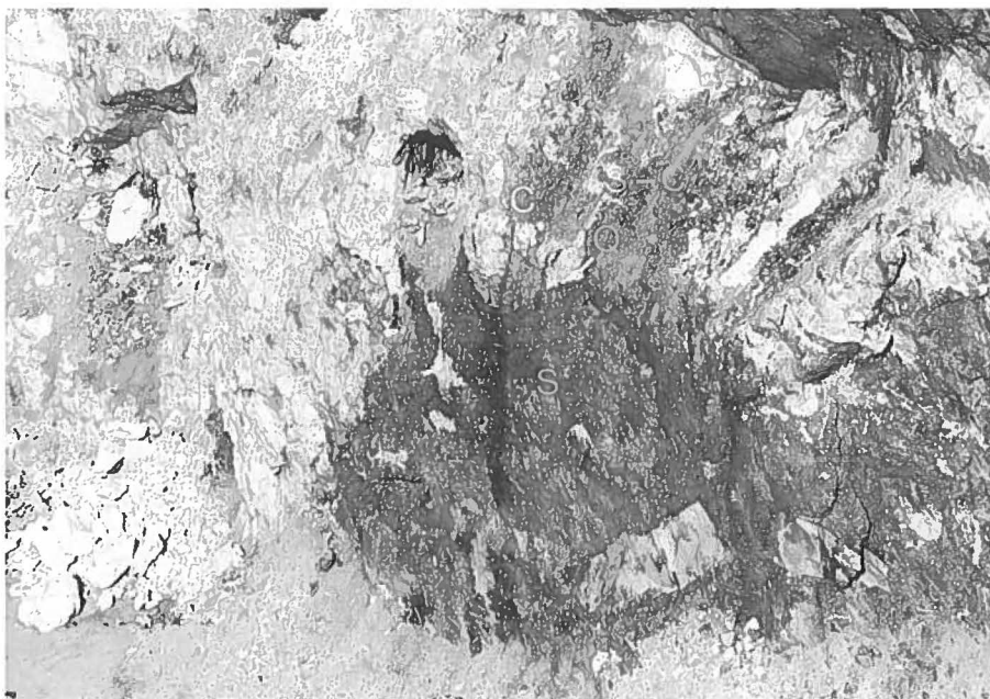
Fig. 14. Upper boundary of the massive siderite unit (S) against pure cryolite (C) and siderite-cryolite (S-C); c. 50 m below sea level, N quarry wall, N end of threshold. The exploration tunnel in the top centre of the photo is 2 x 2 m. Note the quartz crystals (Q) resting on the massive siderite.
