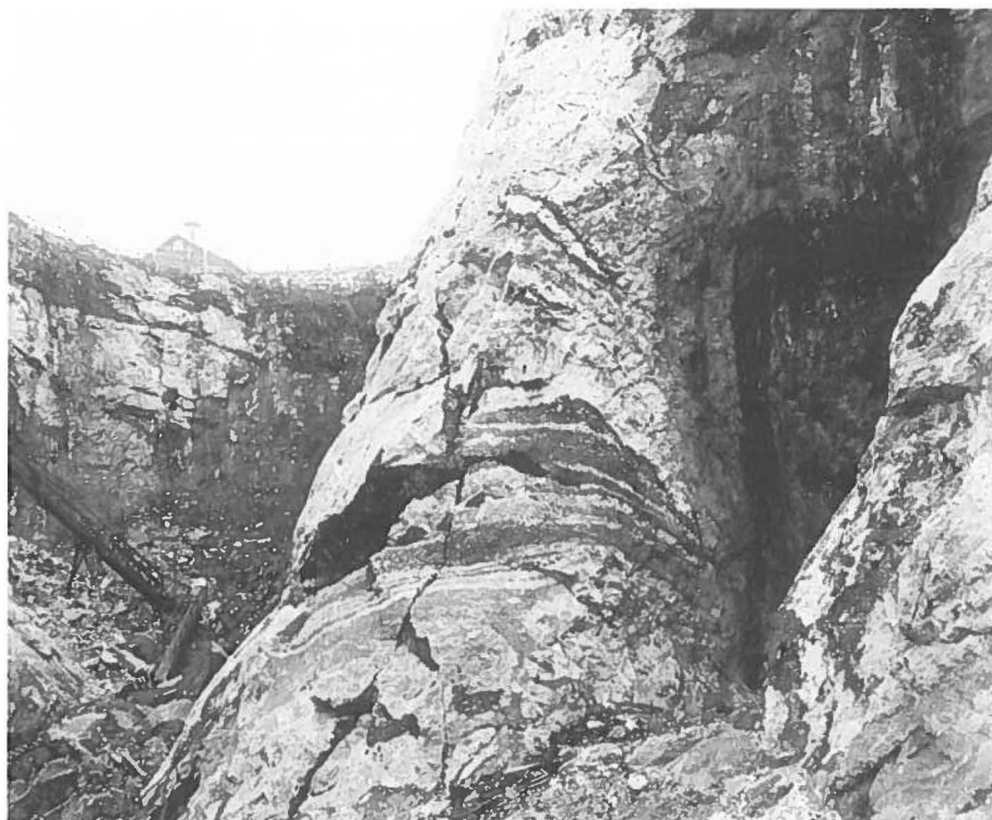
Fig. 8. Irregular banding near the eastern margin of the deposit at the base of the siderite-cryolite unit; c. 30 m below sea level, SE part of the quarry. This pillar (no. 2 of the old workings) is c. 6 m wide. Photograph by R. Bøgvad 1932.
