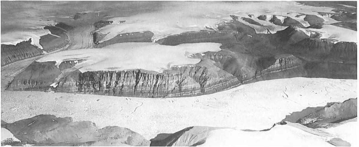
Fig. 3. View eastward across J. P. Koch Fjord showing Gustav Holm Dal between the two ice caps in the middle distance. Perssuaq Gletscher lies to the left. The cliffs along J. P. Koch Fjord are in excess of 1 km high and exhibit a mainly carbonate sequence extending from the Lower Cambrian to the Middle Ordovician (Photo: Geodetic Institute, Copenhagen).
