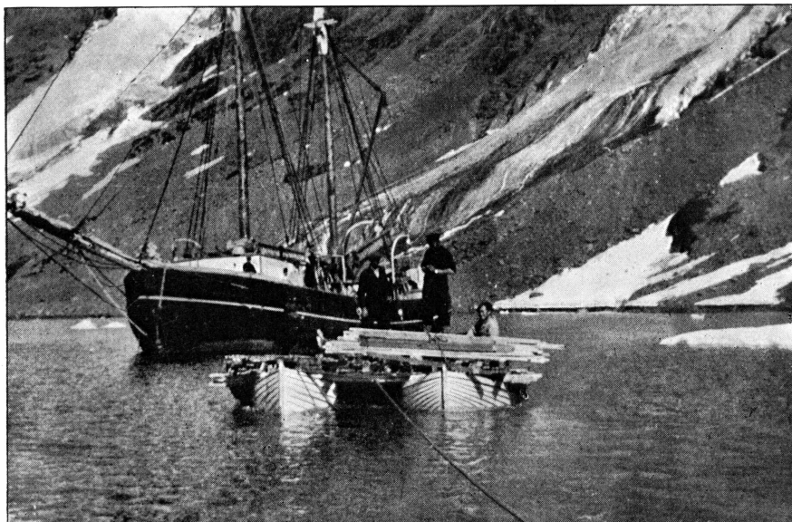
Fig. 20. Transport of building materials in Uttental Sound.
