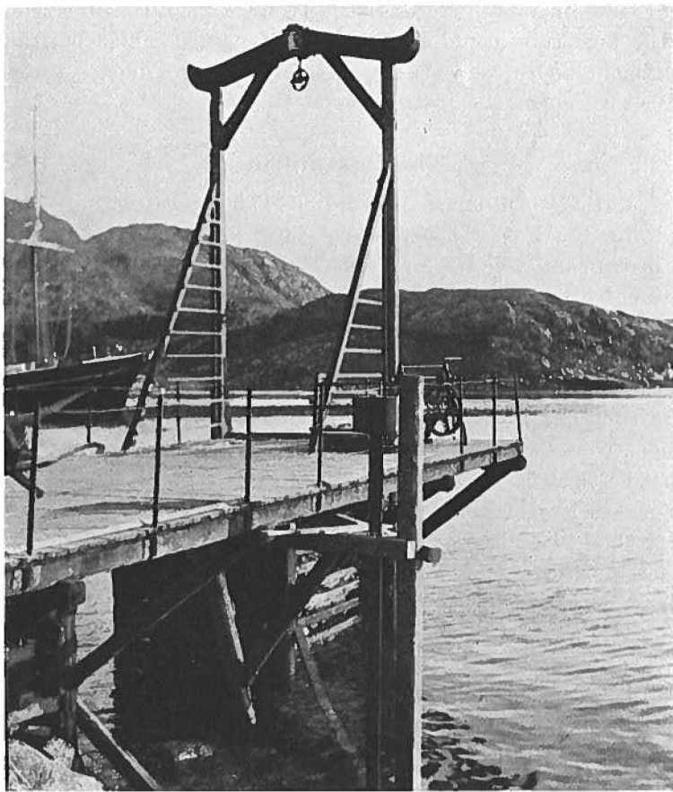
Fig. 4. The picture shows the jetty in Julianehaab harbour, with the extension on the south side. Inside the heavy perpendicular post is seen the float-tube (marked below with ↑) which carried the instrument at the top, covered by a square box.
