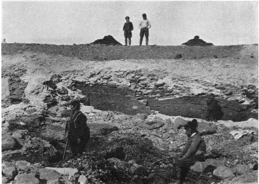
Fig. 5. The coal mine in the coast section at Ikalissat. The coal bed is seen in the lower part of the figure, partly hidden by small heaps of mined coal, and covered by a rather solid bed of coarse sandstone.
