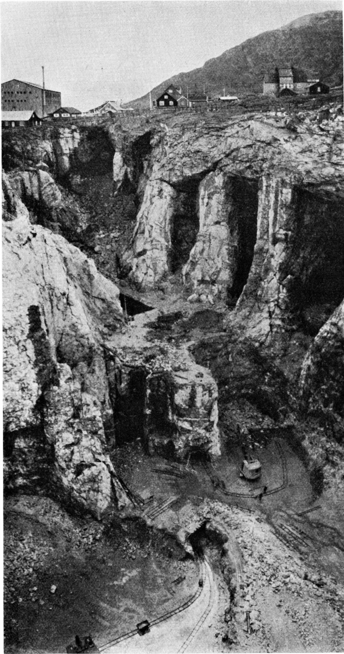
Fig. 1. View of Ivigtut Cryolite Quarry, looking east (autumn 1937). In the left foreground, the foot of the elevator pillar, and, to the right of this, the entrance to the lower tunnel flanked by the area from cote —55 to —60. Above the excavator to the right, the western part of the eastern quarry.
