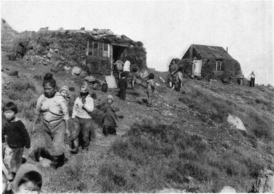
Fig. 28. Two types of modern houses at Angmagssalik; to the left a house built of sods, to the right one constructed of framework and boards.
