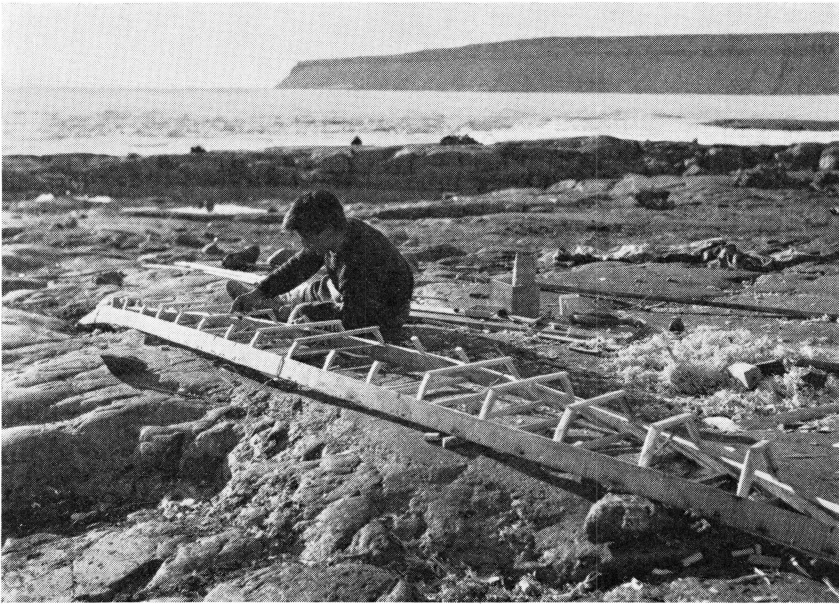
Fig. 56. Qarqutsiaq's kayak under construction
