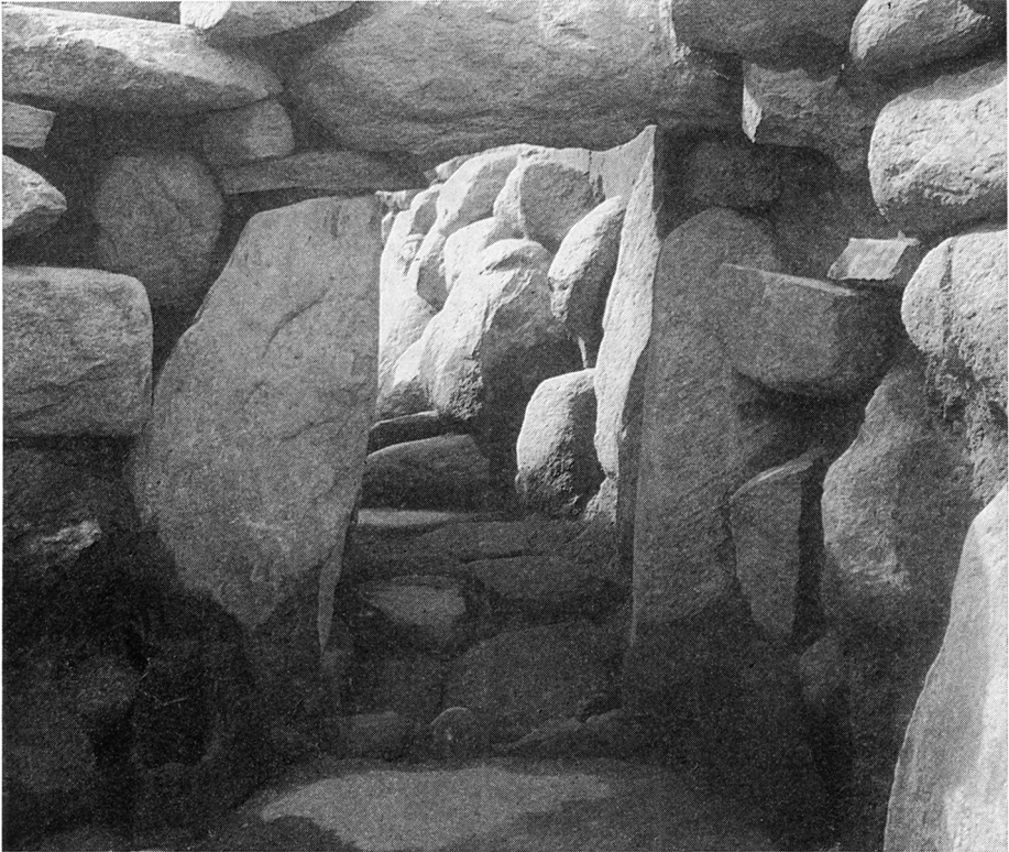
Passagen mellem kammer og gang i kælder G på Løgten Mark, set fra kammeret. De to svære stolper, der ses på begge sider af indgangen, må have tjent som dørramme, den ene dog eventuelt samtidig som sule. The passage between chamber and corridor in Cellar G at Løgten Field, viewed from the chamber. The two massive posts on either side of the entrance must have served as doorposts, though one may also have been a roofpost.
