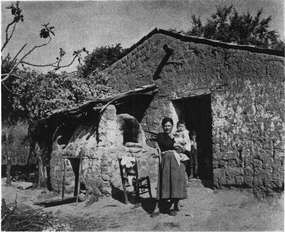
Fig. 1. Markhus i Sartano med tilbygget bagerovn. Under ovnen stald. HR fot. 1955. Country house at Sartano with lean-to baking oven, and pen below the oven.
