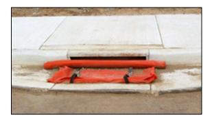
Figure 6: Catch basin for erosion control maintenance
