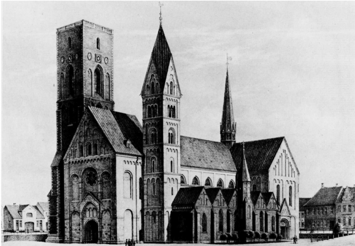
Fig. 2. The Cathedral from the south-west, with the apse, the transept and nave of the 12th–13th century. The outer naves were added in the 14th and 15th century, the Great Tower shortly after 1300. From a drawing by Harald Bruun 1906, after conservation works 1904 by H.C. Amberg. Photo: The National Museum.
