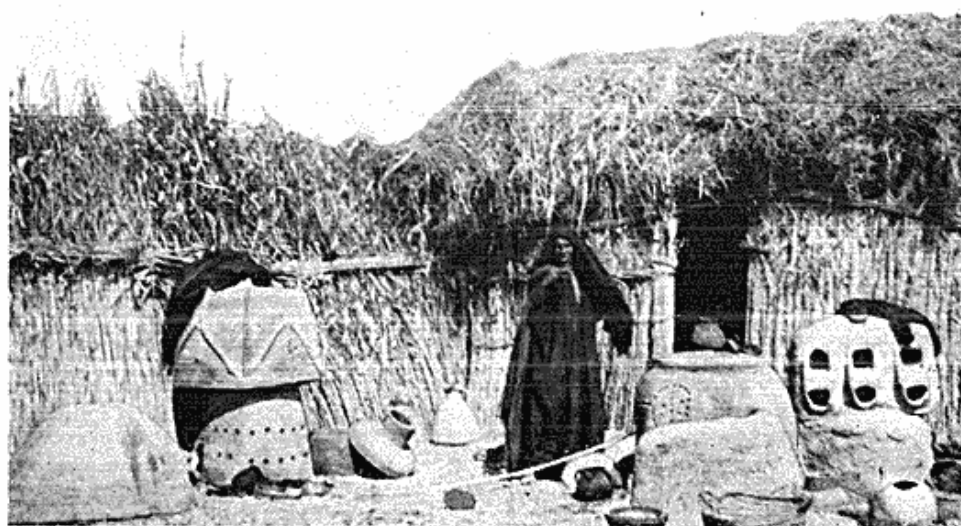
Fig. 2. INSIDE THE EZBEH. Cottage for the spring in the open field, constructed of doorrah-stalks tied together, and only in the corner a small place covered with a roof as room for the night. The furniture is made of clay and mud mixed with dung from camels and donkeys.
