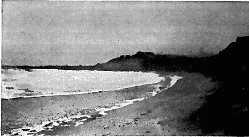
Fig. 5. Leaside Erosion on the Southside of a Group of Groins at Bovbjaerg, North Sea Coast, Denmark.
