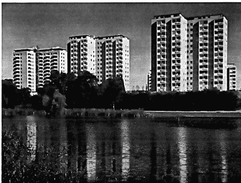
Fig. 5. The "point blocks" at Bellahøj, built in the 1950's.
