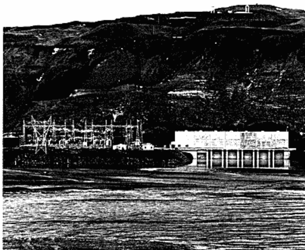
Fig. 1. Búrfell vandkraftanlæg (210 MW) i Thjórsárdalur, Syd-Island. Fig. 1. The Búrfell hydropowerplant (210 MW) in Thjórsárdalur, South Iceland. Photo: S. Thorsteinsson.
