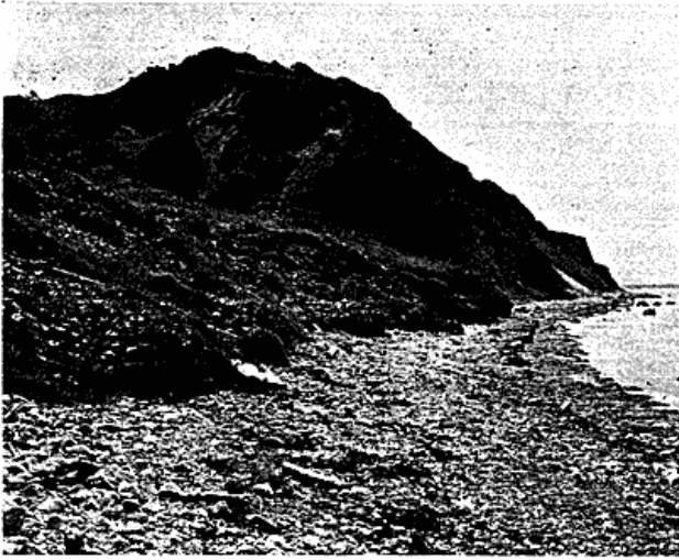
Fig. 10. The toe area of a mudslide which has been trimmed by recent marine erosion.
