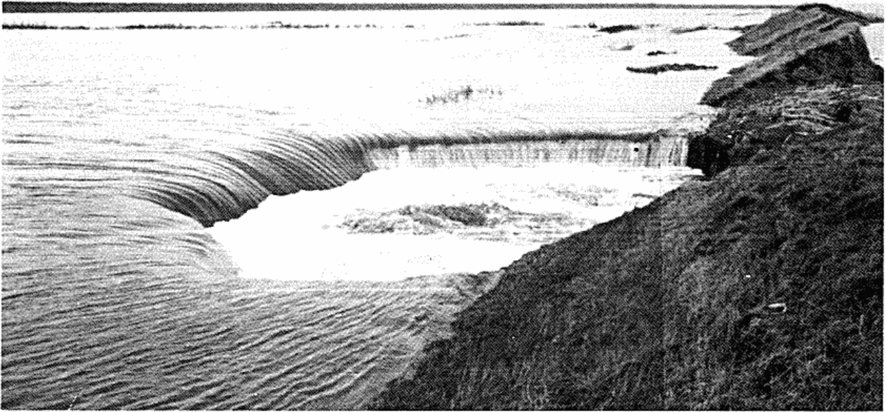
Fig. 12. The area between the old and the new Juvre Dike after the storm surge in 1981. The trapped water has breached through the dike and flows out into the Juvre Priel forming a cascade.
