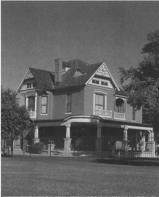
Petersen House Museum i Tempe i Arizona.
