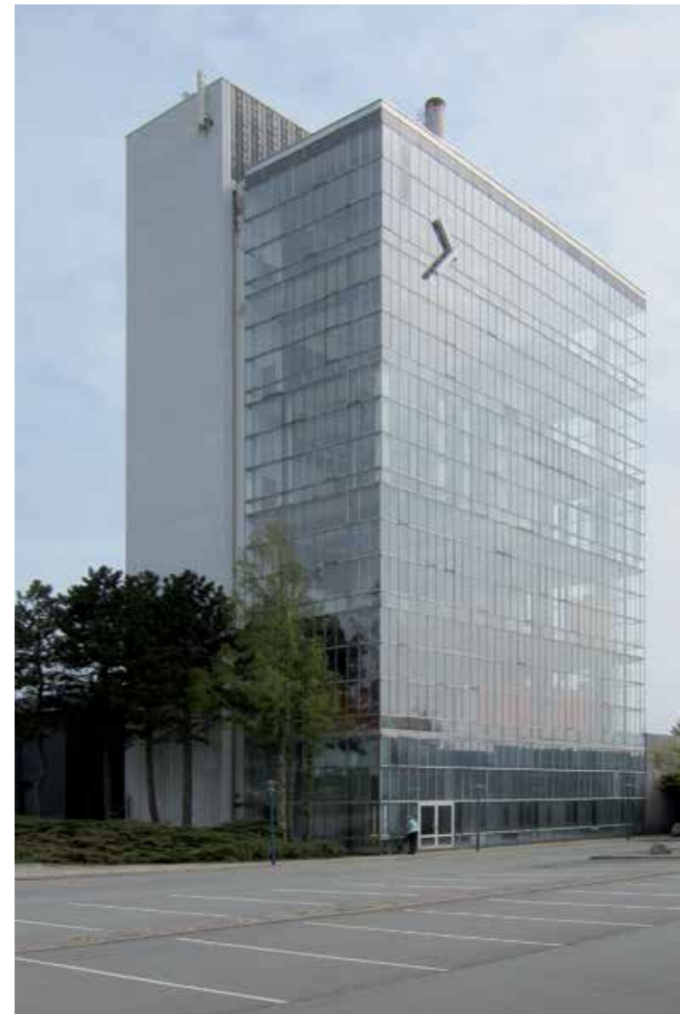
Irma Kafferisteri – coffee roasting plant, built 1967 and listed without machinery in 2014. Photo Slots- og Kulturstyrelsen 2014.
