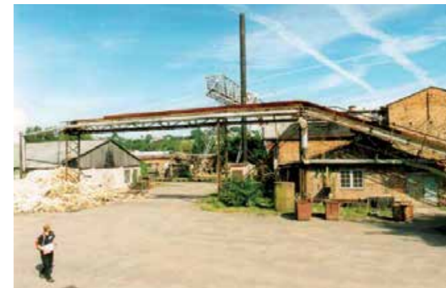
From the left: storage, pile of used billets, conveyor, boiler house. In the background: trestle crane.
