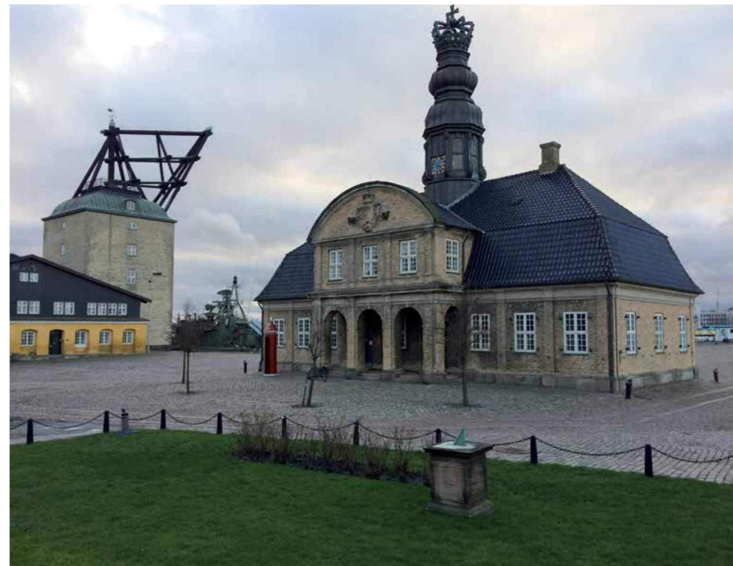
The Naval Dock Yard, Copenhagen, the Rigging Shears of 1750 and the Guard Building of 1745, both listed in 1918. Photo CAJ 2020.
