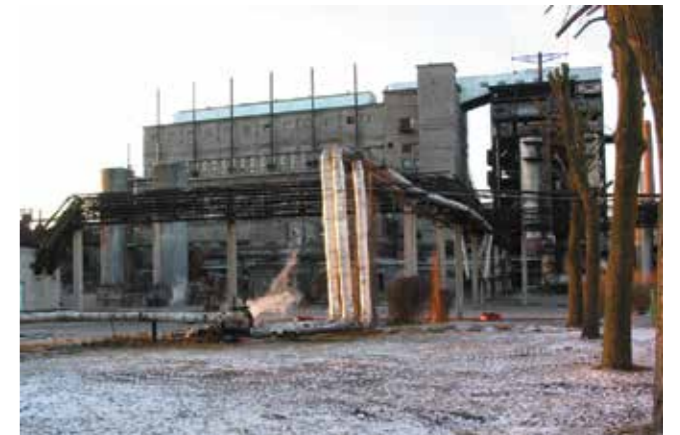
One of the shale oil workshops from the soviet period in Kohtla-Järve Estonia, run by the Viru Keemia Grupp, which focus on oil shale mining, shale oil, combined heat and power production. Photo CAJ November 2002.
