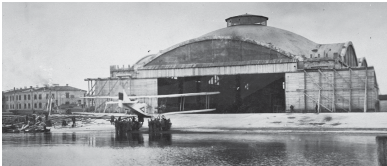
An extraordinary engineering achievement, the Tallinn seaplane hangars was completed as part of the unfinished giant project of the Tallinn military port of the Russian Empire in 1917 according to the project of the Danish company Christiani & Nielsen. Photo: 1920s. Estonian National Archives photo collection EFA.II4.A.335.365
