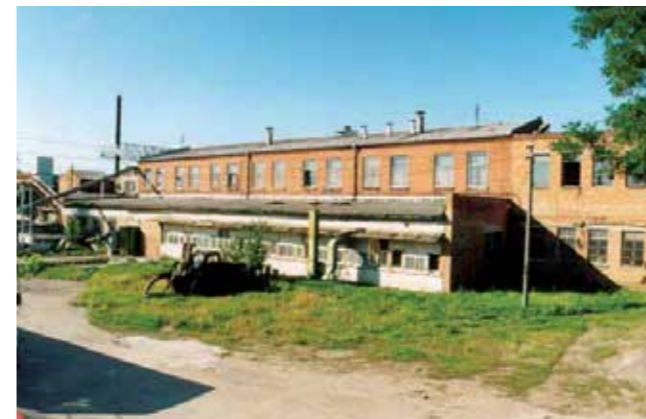
Match production building, S facade with loading ramp.
