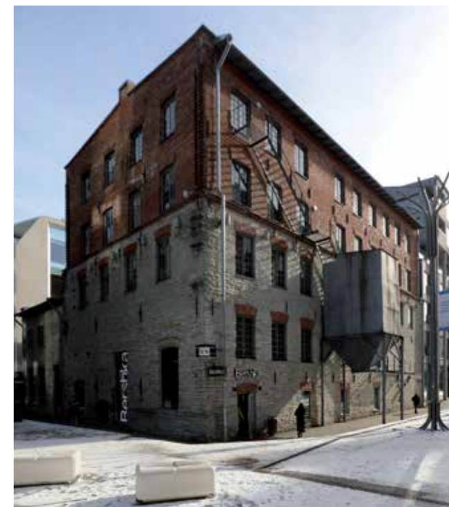
The barley mill (1905) of Roterma factories burned out in 2000 and was restored by 2007 (Teigar Sova Arhitektid). Photo: Henry Kuningas 2022
