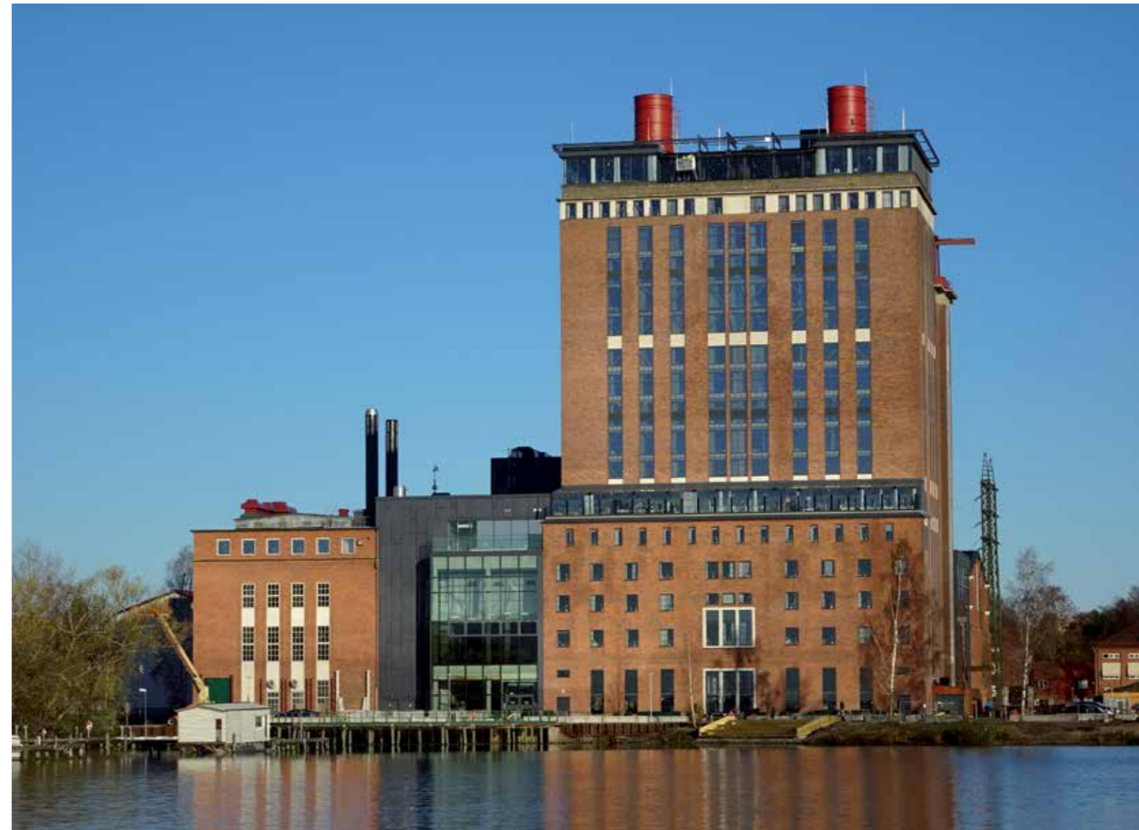
The steam power plant in Västerås (Ångkraftverket Västerås), Photo Dependability, 2017, Wikimedia commons, CC BY.
