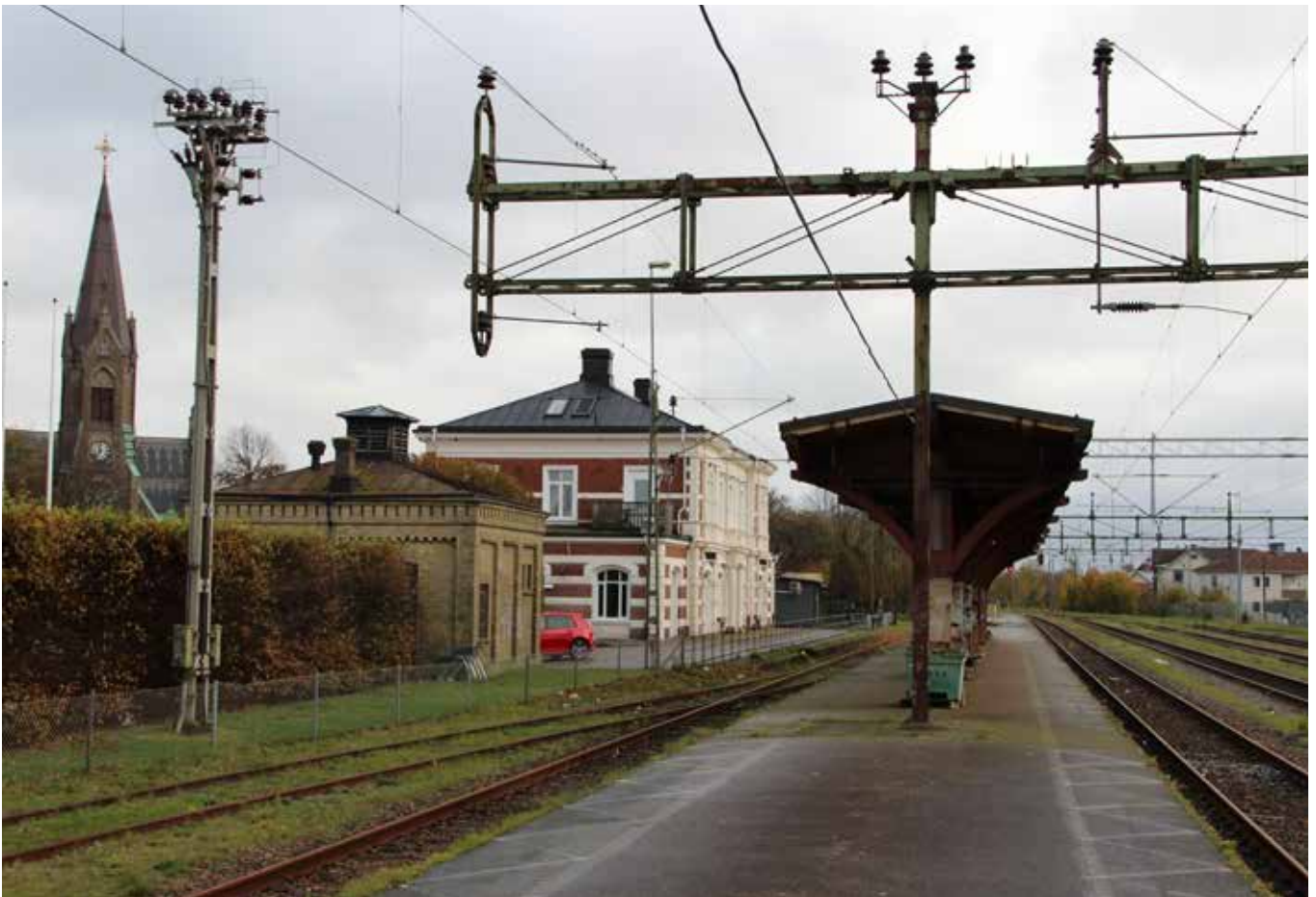
Falkenberg railway station, nowadays closed. The curved platform canopies (1920s) and the catenary system (1930s) are typical for the Swedish State Railways. H. Ranby 2023.
