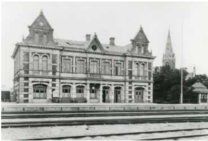
Central Halland Railway. Falkenberg railway station, designed by A. C. Pettersson. In this picture with its original decorative gables. Swedish Railway Museum.
