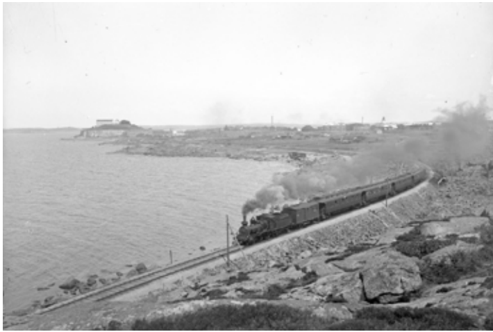
Central Halland Railway. The line at the Varberg Fortress. Swedish Railway Museum.
