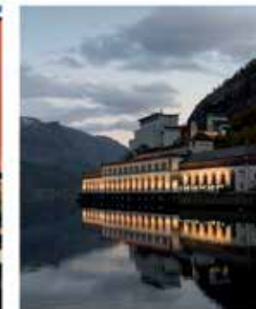
Tyssedal Hydroelectric Power Station Photo: Harald Hognerud, NVIM
