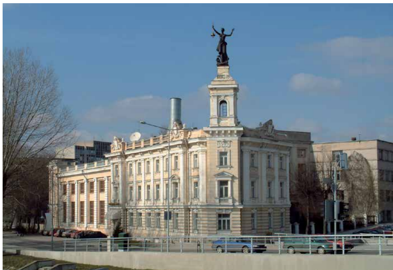
The first public power plant in Vilnius (1903), listed and converted to the Museum of Energy and Technology in 2003: Marija Drėmaitė, 2004.
