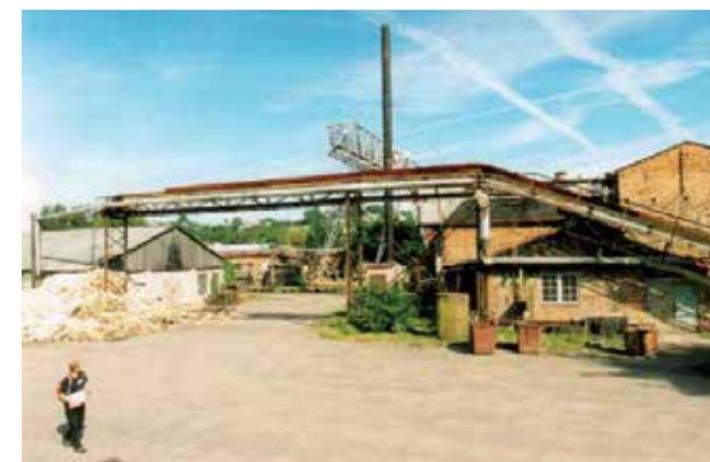
From the left: storage, pile of used billets, conveyor, boiler house. In the background: trestle crane.
