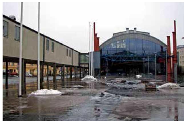
Former Rope Factory in Turku was converted into a conservatory and art academy in the 1990s. Foto: Timo-Pekka Heima/Finnish Heritage Agency 2007.
