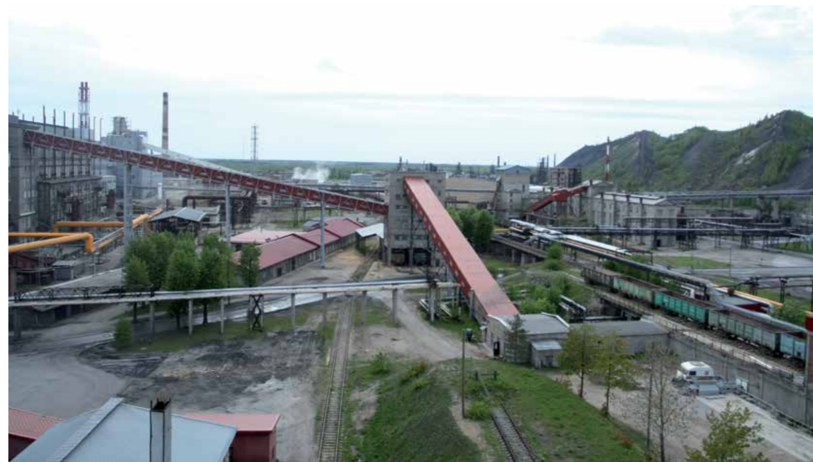
The first factory of the state-owned Kohtla-Järve oil shale factory was completed in 1924. The continuously operating factory grew into the largest oil factory in Estonia during the Soviet period. Photo: Henry Kuningas 2011
