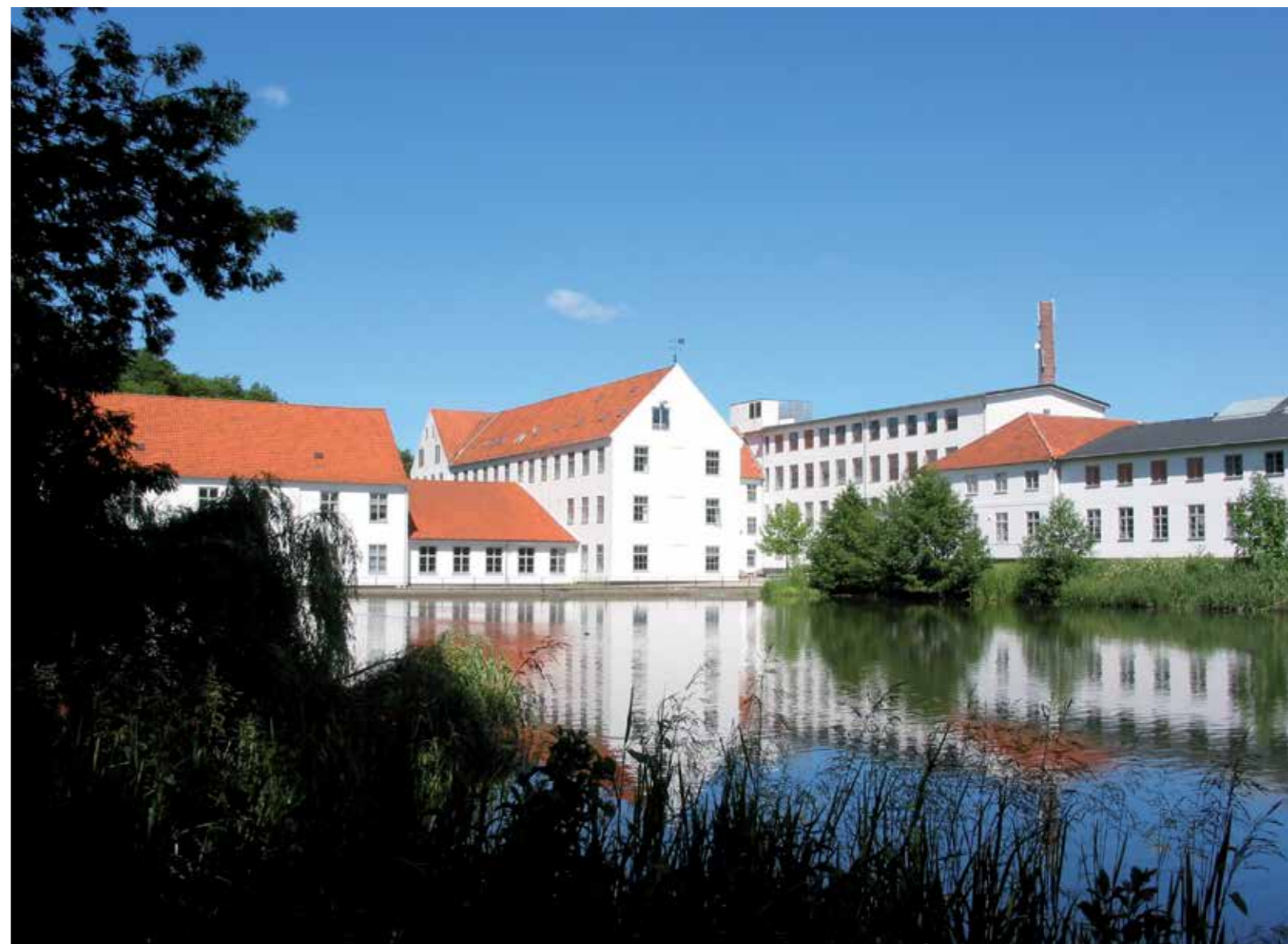
Usserød Klædefabrik – Textile Mill, built 1803-1950 and listed 1982. Photo CAJ 2003.
