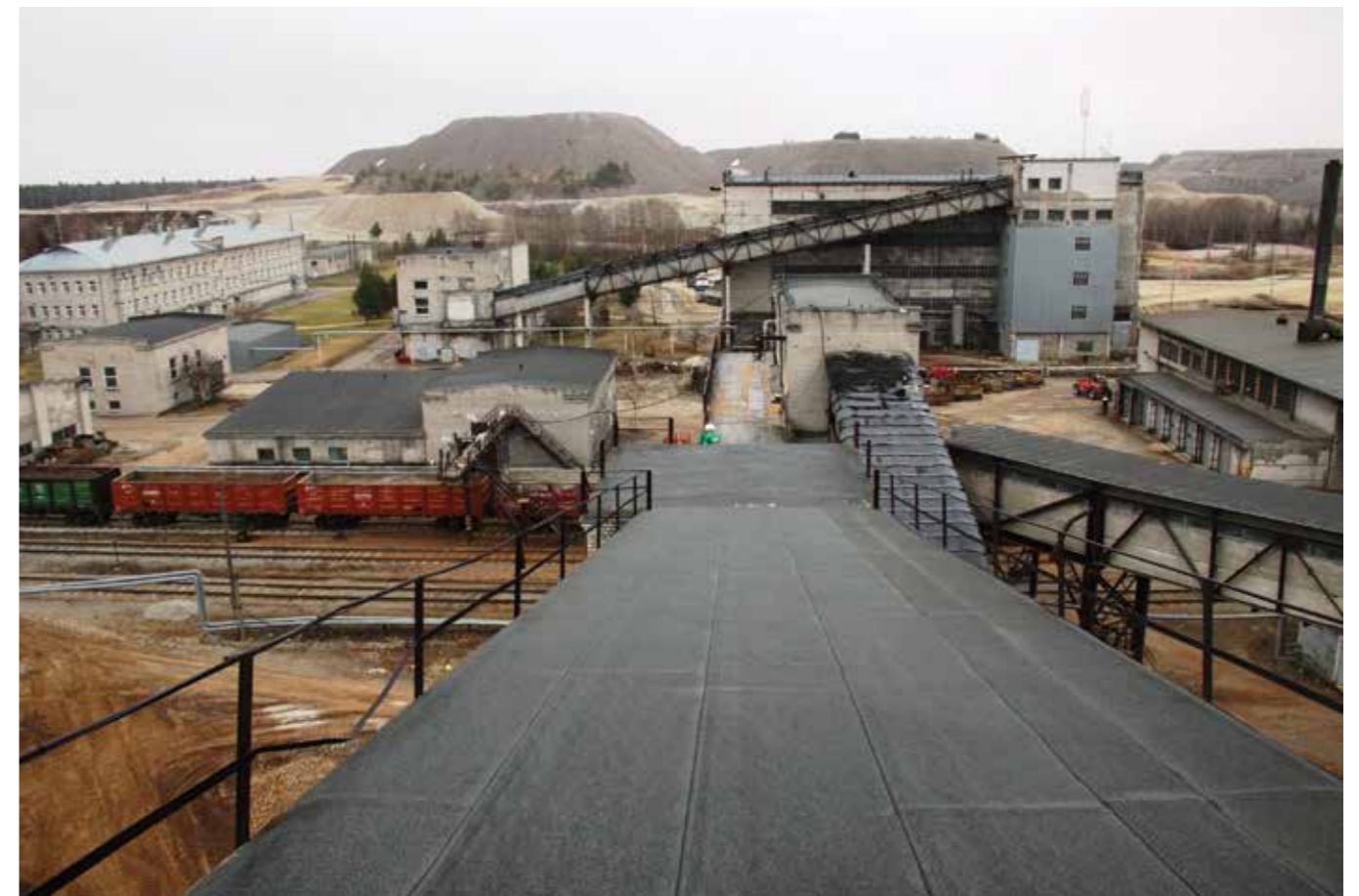
13 During the 20th century, Estonia was the world’s largest oil producer through extraction in oil shale mines, a production that began in 1921. From 1924, oil shale was used to generate electric power, but the oil gained importance above all after conversion to gas for industrial companies and households in Estonia and in Leningrad. The increased need for electricity in the north-western Soviet Union soon led to the construction of large oil shale-fired power plants. A mining centre was Kohtla-Järve in the northern part of the country. Here, extraction reached its peak in the 1980s. Since then, mines have been closed, dilapidated or turned into museums. Today, Viru Keemia Grup, a private Estonian large-scale industrial company in Kohtla-Järve, conducts oil shale mining, combined with heat and power production as well as production and marketing of fine chemical products. Estonia still has the two largest oil shale-fired power plants in the world. In recent years, production has decreased due to the large emissions of greenhouse gases and of waste that destroys the environment. Photo: Henry Kuningas 2013.
