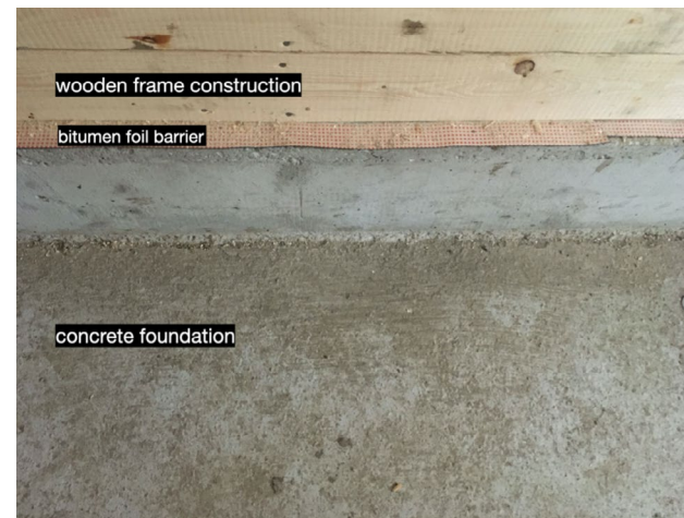
Figure 2: The wooden frame construction sitting on the concrete foundation
