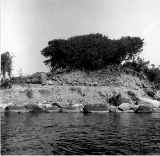
Figure 5. The cleaned section in the coastal cliff, showing the most threatened part of the dolmen Damsbo Skjoldmose on Funen, 1984. Photo: J. Jeppesen.
