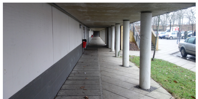
Fig.11 The residential block before renovation..
