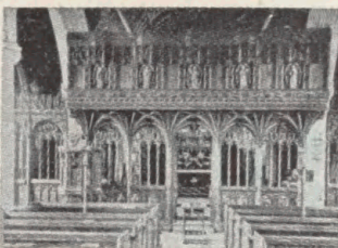
KENTON. The chancel screen and roof loft
