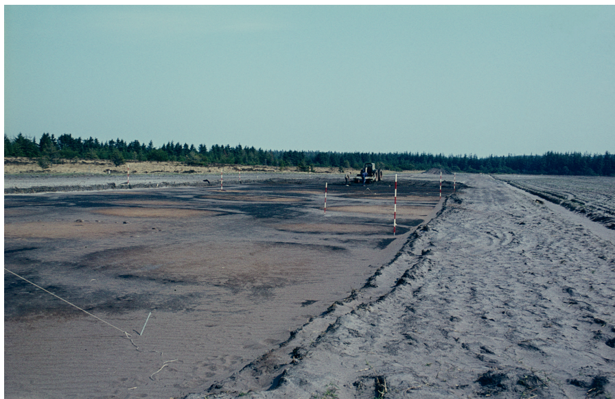
Fig. 4. Jordsluffen i brug ved Aarupgaard. I baggrunden ses det fredede hedeeareal. Fig. 4. Long metal chains pulled by a tractor removed the topsoil at the excavation site. The protected heath area can be seen in the background (photo: E. Jørgensen, 1970).
