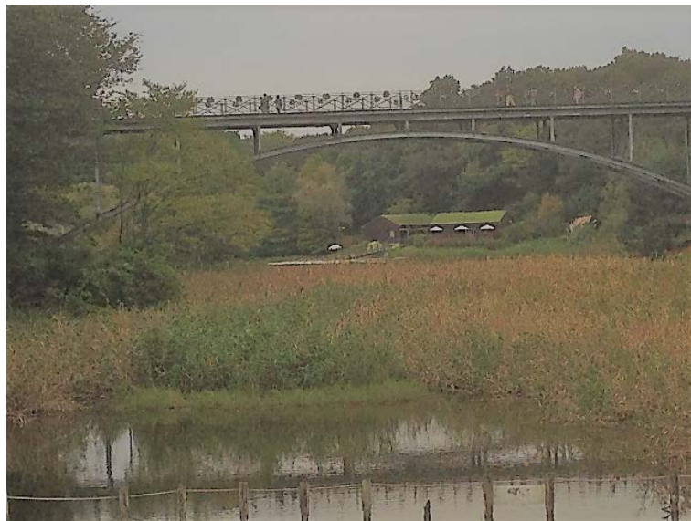
Fig. 11. Iron bridge seen from below. Photo by Kwok-kan Tam.
