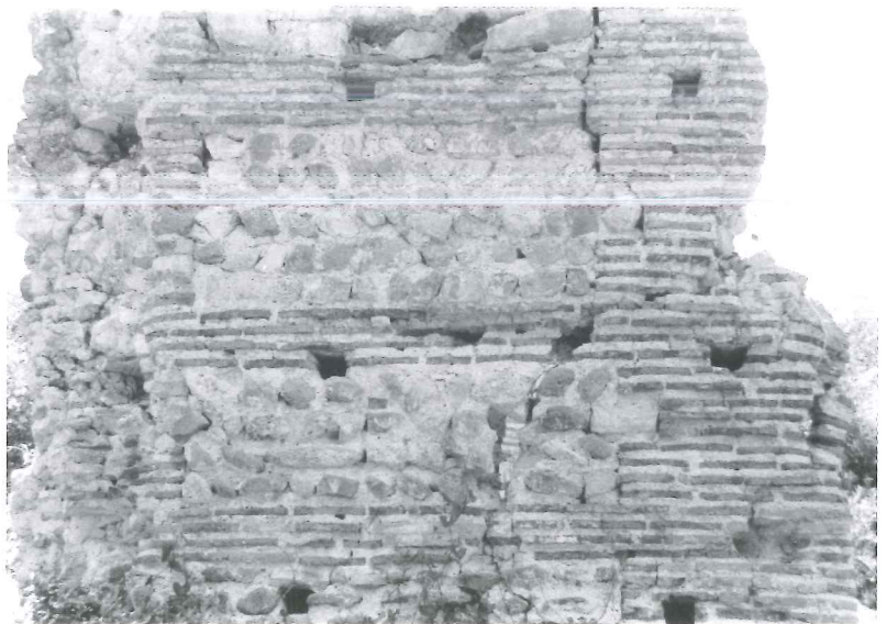
Fig. 4. Riza. Decagon. Building technique (opus mixtum).
