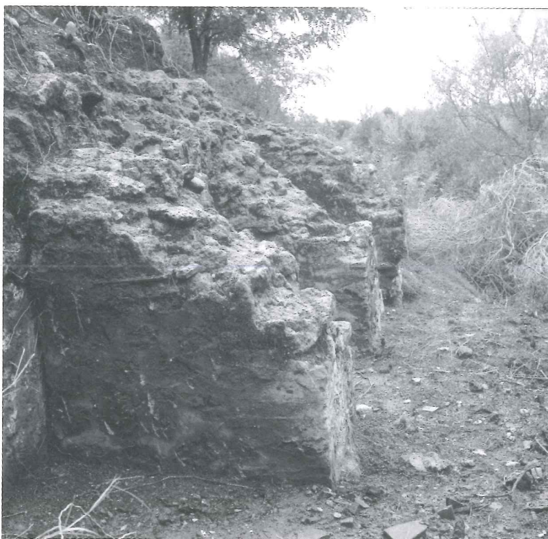
Fig. 6. Agia Pelagia. The wall on the west side of the monastery.
