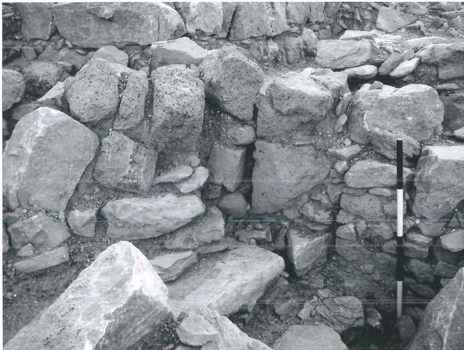
Fig. 10. House C.8, fallen quoins at northwest corner.
