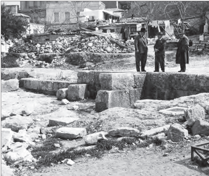
Fig. 60 Zea, Group 1, Phase 3, upper ends of Shipsheds 16, 17(η) and 18(χ) (right). From south-west (commissioned by I.A. Meletopoulos ©Piraeus Historical Archive).
