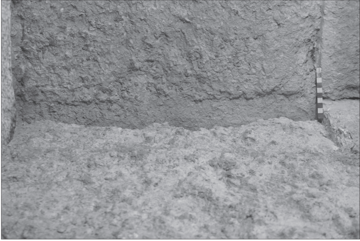
Fig. 74 Zea, Group 1, Phase 3, detail of Spur-wall block C17/18:4 tying into Back-wall section 2a. From north-west (M.M. Nielsen ©ZHP 2006).
