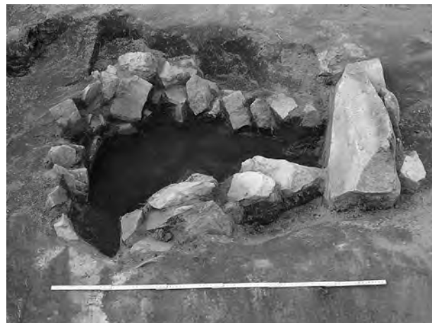
Fig. 8. Buttress foundation at the northeastern side of the church, looking west. Photo: Orri Vésteinsson 2006.
